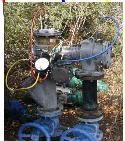
Setting up Test 2 on a Febco RPZD
